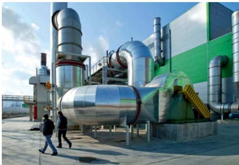
Co-gen plant consisting of 2x 7.5 MW gas turbines integrated with TM 2 (to the right).
