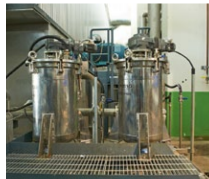
Metso's OptiScreen RF screens provide clean and even starch and coat application.
