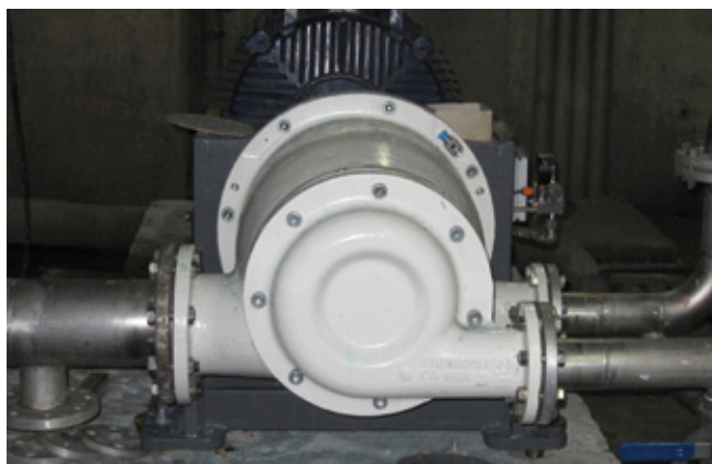
OptiFiner Pro on deinked pulp for trim refining/deflaking at Koehler Greiz GmbH & Co. KG in Germany.
